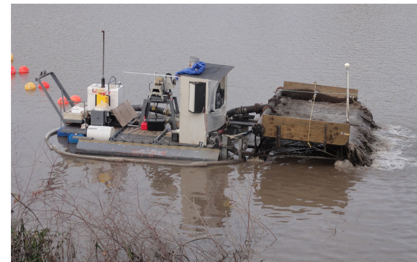
Spreader table used to create thin layer cap
