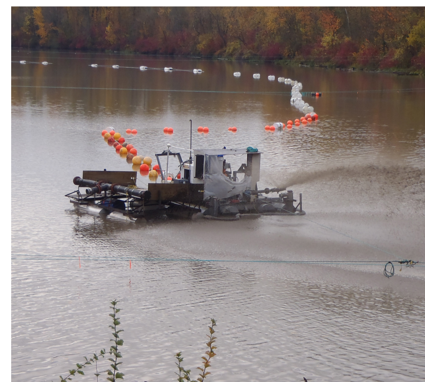
Sand cannon used to disperse sand for thin layer cap
